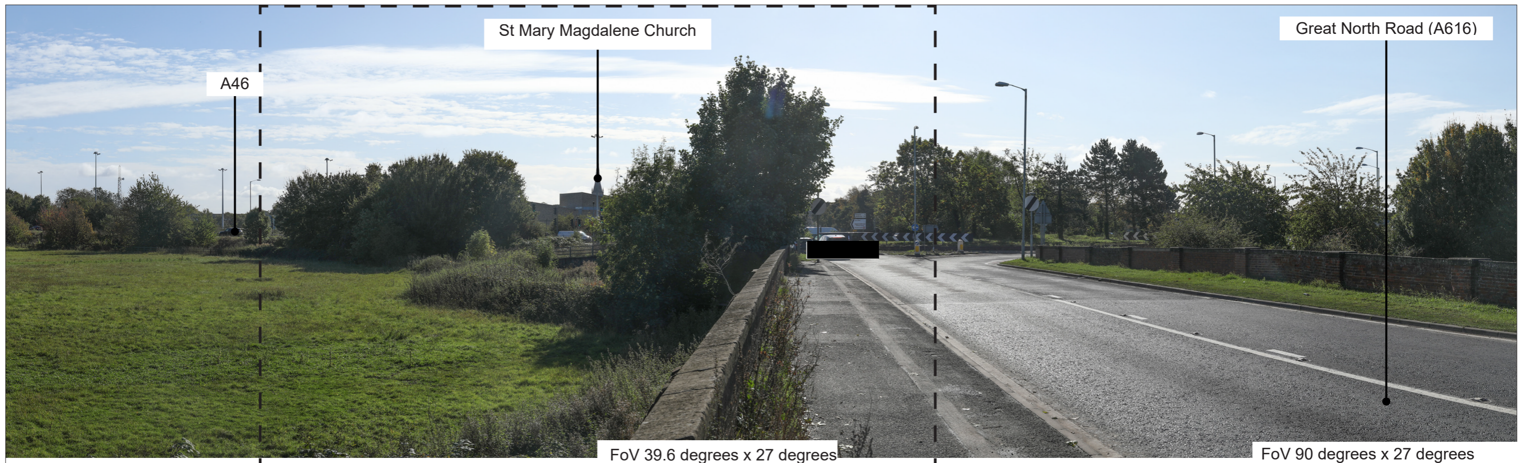
Photomontage 25: Existing view (cylindrical projection, field of view 90 degrees x 27 degrees, to be viewed at A1)
