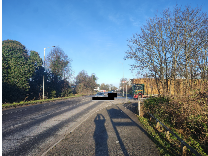
Existing view north towards Cattle Market Junction
